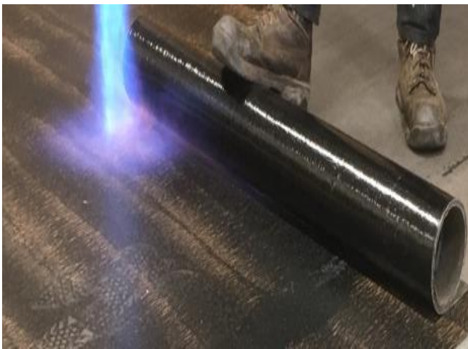
Figure 3 - Typical torch on method of application
